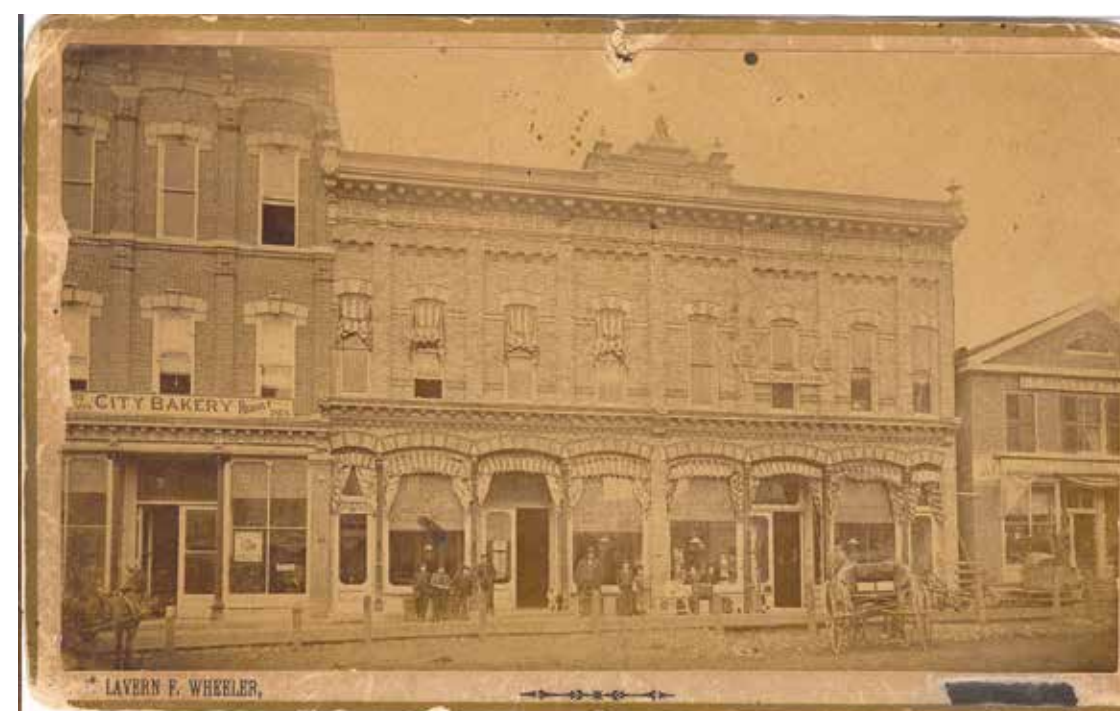
Figure 2 – View of Rehfuss and Kapp Building (left), and the 1837 William Carr Brick Building on Exchange Place (right)
